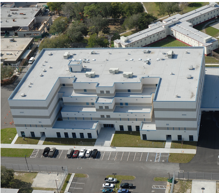
Pinellas County Jail, Healthcare Facility Expansion Clearwater, FL
