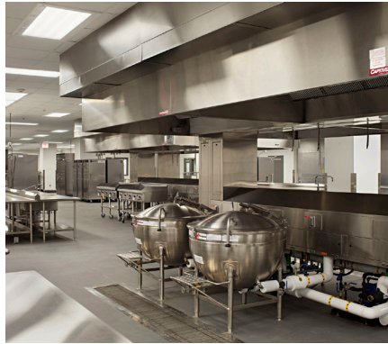
Wake County Detention Center: Phase 2 Expansion Raleigh, NC
