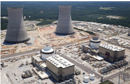
Vogtle Nuclear Power Plant Units 3 & 4
