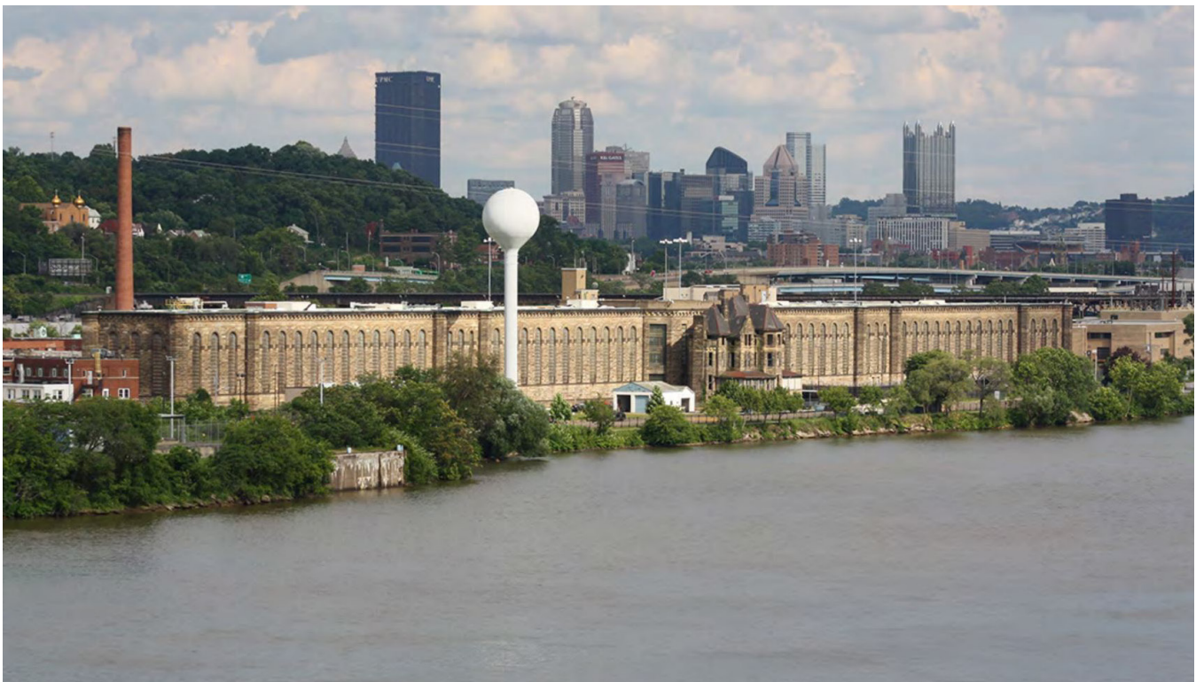
SCI-Pittsburgh, front facade, looking southeast, showing the close proximity to the Ohio River in the foreground and Downtown Pittsburgh in the background (Sources: Charles Rosenblum, PHMC National Register Nomination Form)
