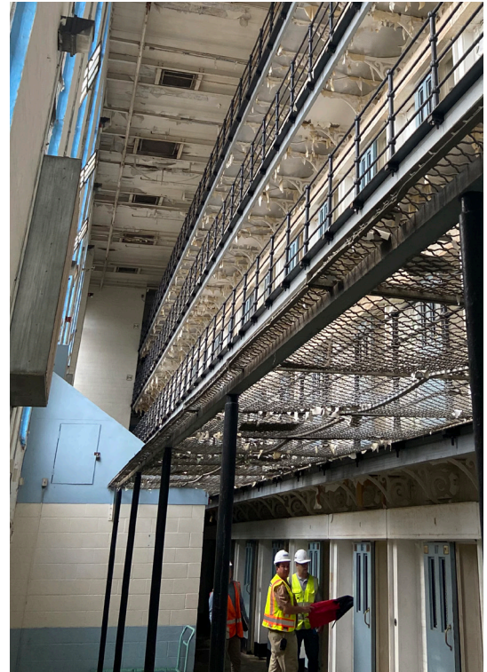
Michael Baker Team Site Inspection, July 2022
