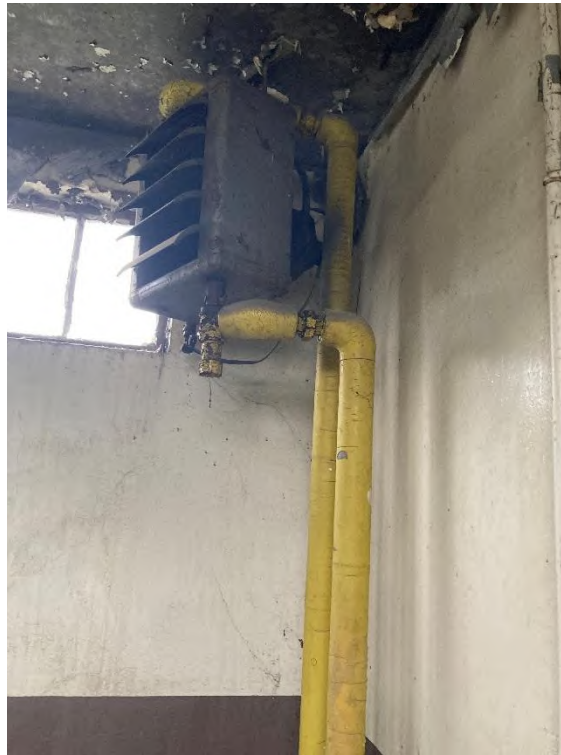
Positive ACM located in thermal pipe insulation in building 31, rooms 1, 2, and 5.
