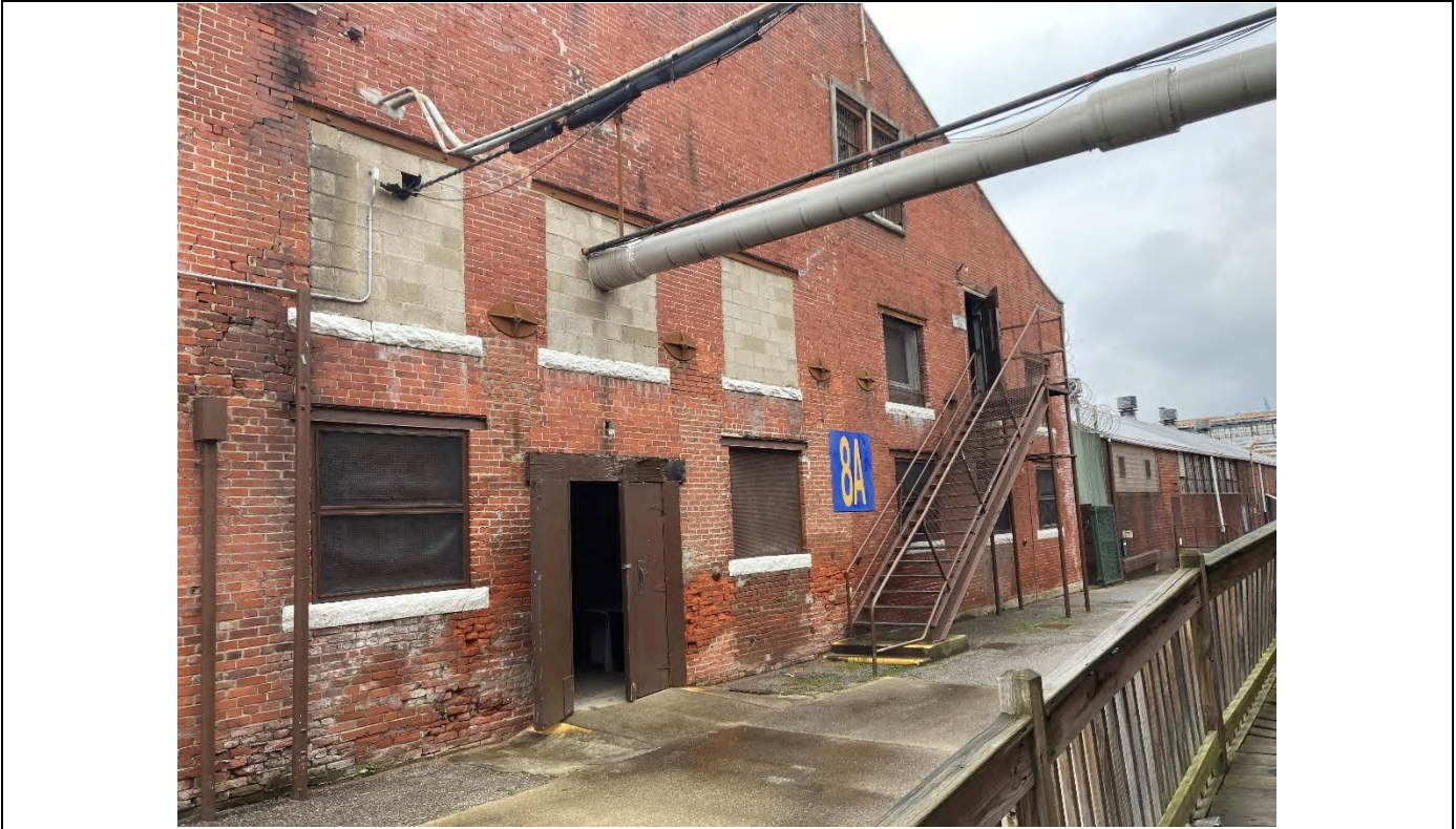
Photograph #1 | SCIP Building 8A – Dietary Storage.
