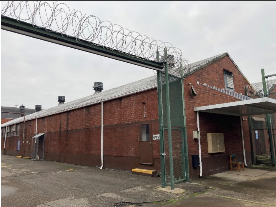
Photograph #1 | SCIP Building 10 – Services Building.
