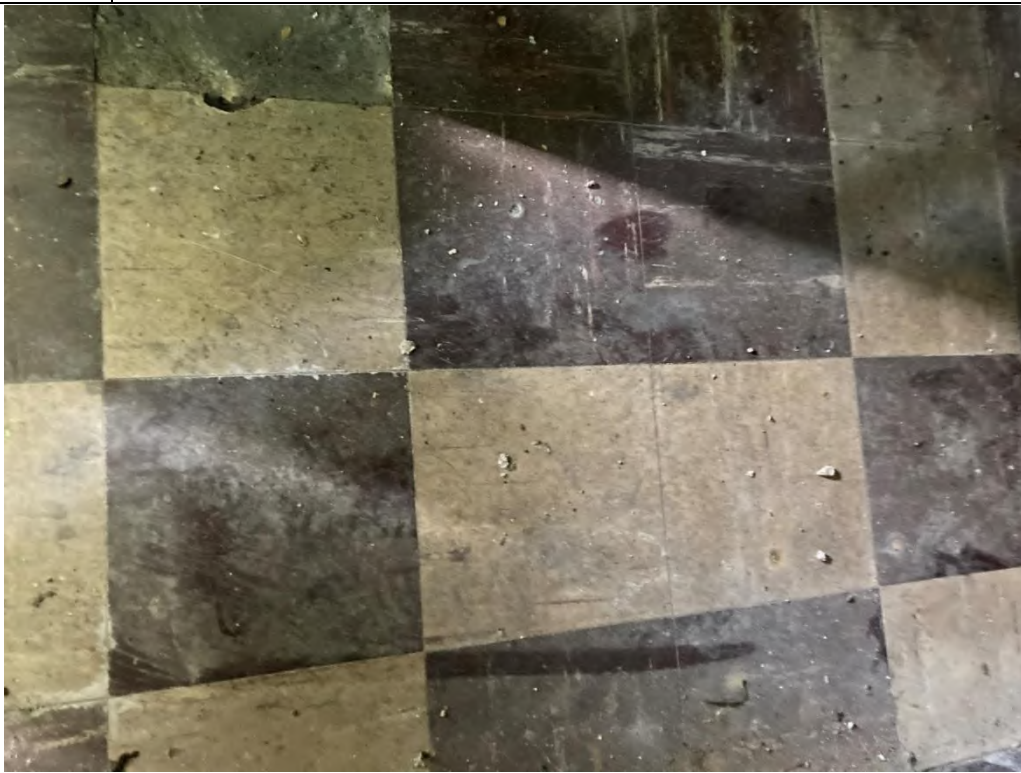
Positive ACM located in 9'x9' white and brown vinyl floor tiles and adhesive located in Building 4.
