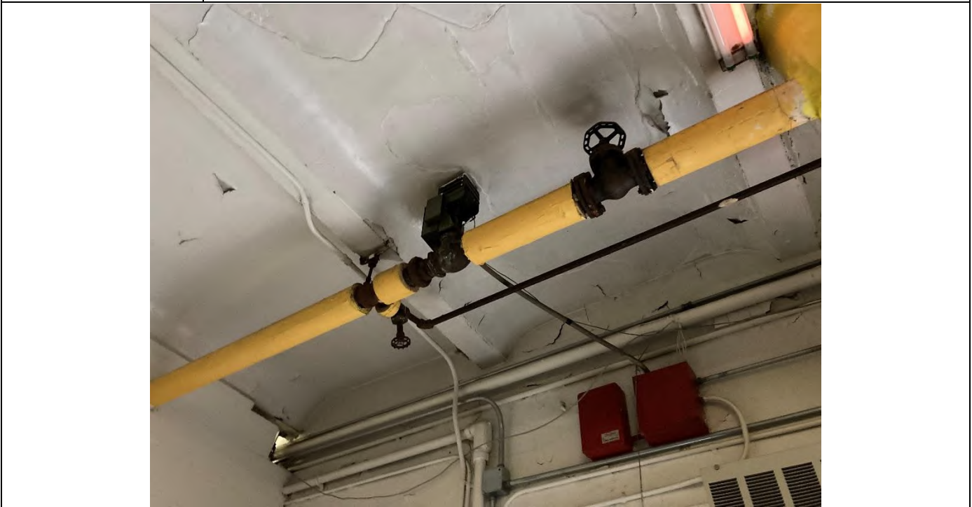
Photograph #2 | Positive ACM located in thermal surface insulation located in building 8A
