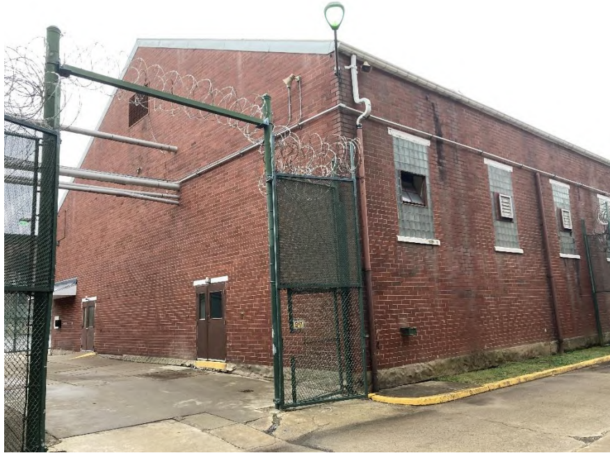
Photograph #1 | SCIP Building 16 – Gym.
