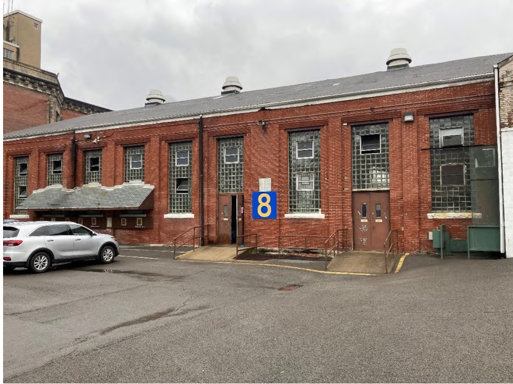
Photograph #1 | SCIP Building 8 – Auditorium.
