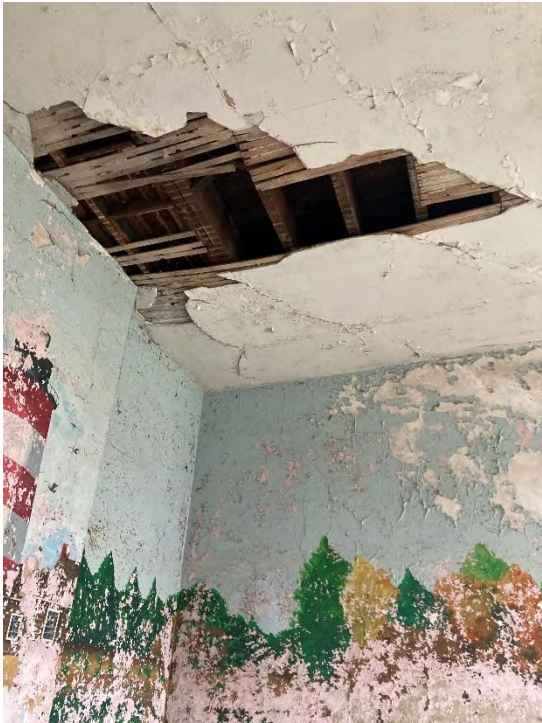
Positive ACM located on the second floor of Building 1 – Front House.
