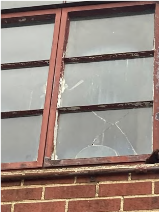
Positive ACM located in window caulk in building 32.
