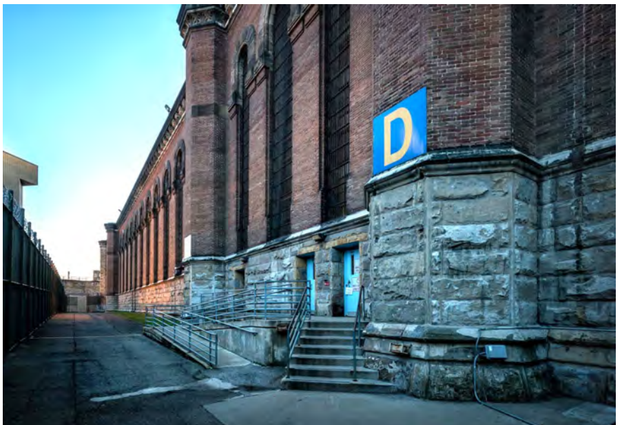
Photo 16. Main Penitentiary Building, east facade, looking south, showing a close up of the stone base of the building and one of the ADA ramps to the housing units.
