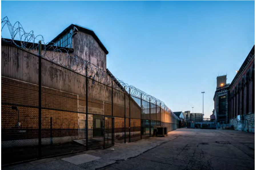
Photo 48. Correctional Industries Shop Building, looking south, showing the Tag Shop (11) at left.
