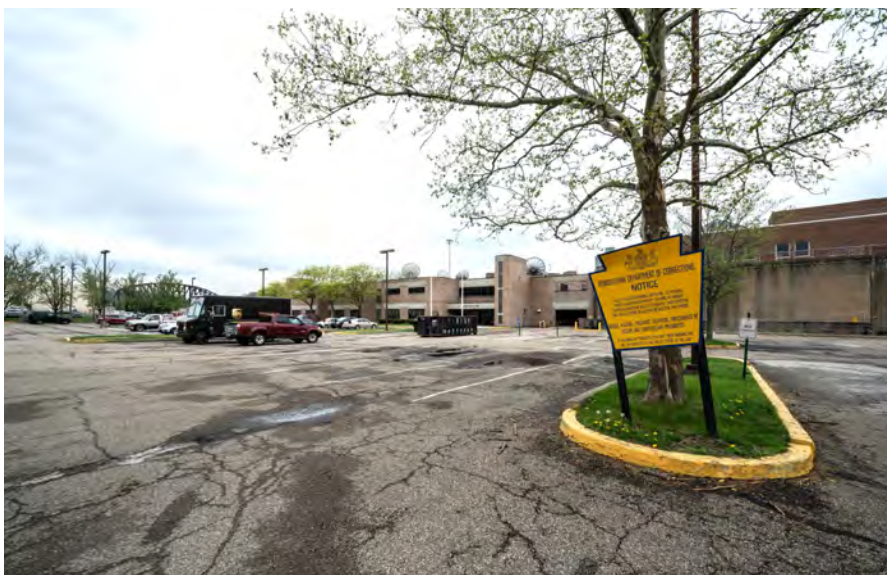
Photo 6. The New Front Yard of the Penitentiary, created as part of the 1984 master plan, looking southwest, showing the Administration and Visitors Complex at center.
