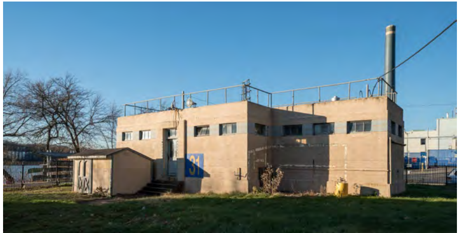
Photo 82. Sewage Pump House, south facade, looking northwest.
