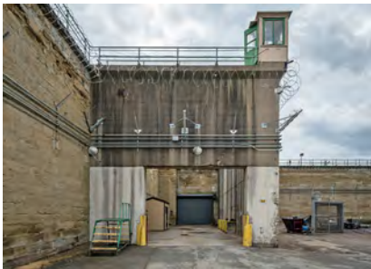
Photo 88. Southwest gate, looking south, showing the cast concrete vehicle Sally Port with guard tower atop.
