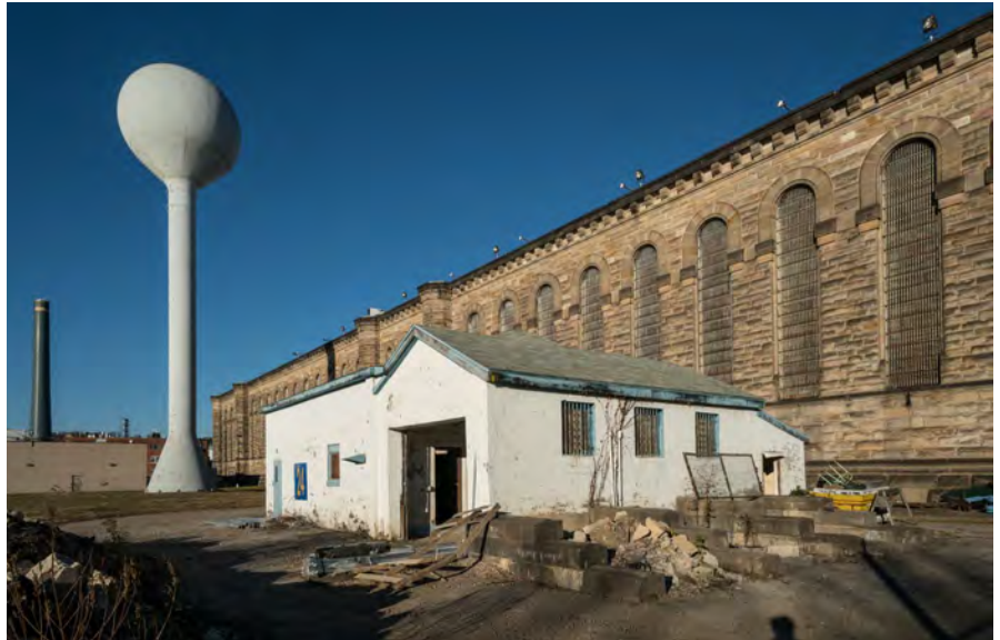
Photo 72. Storage Building, looking northeast, showing the former garage of the Warden's Residence with the North Wing of the Main Penitentiary Building and water tower in the rear.
