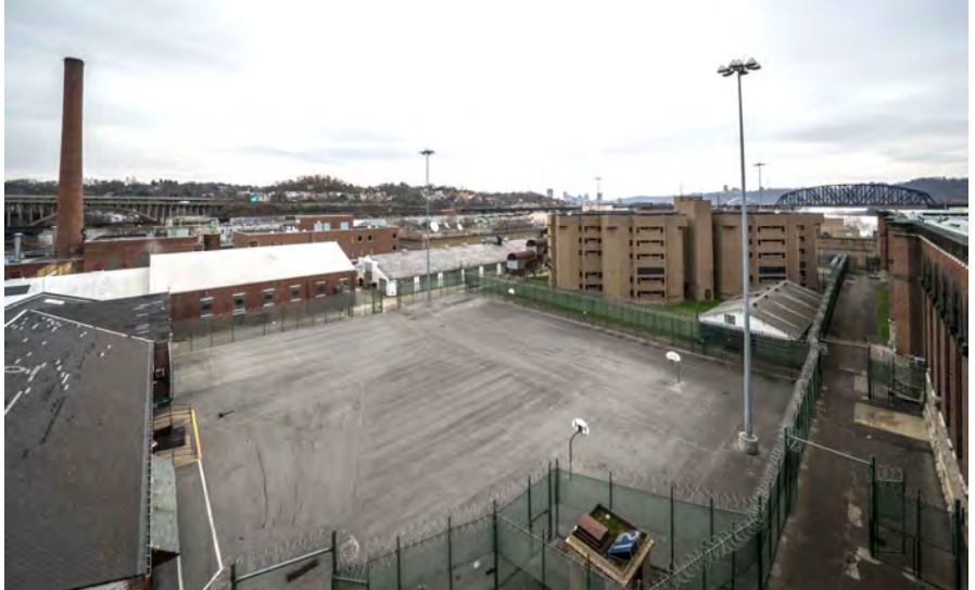
Photo 5. South end of the Secure Perimeter, looking southeast from the roof of the Rotunda, showing the Main Yard (center).
