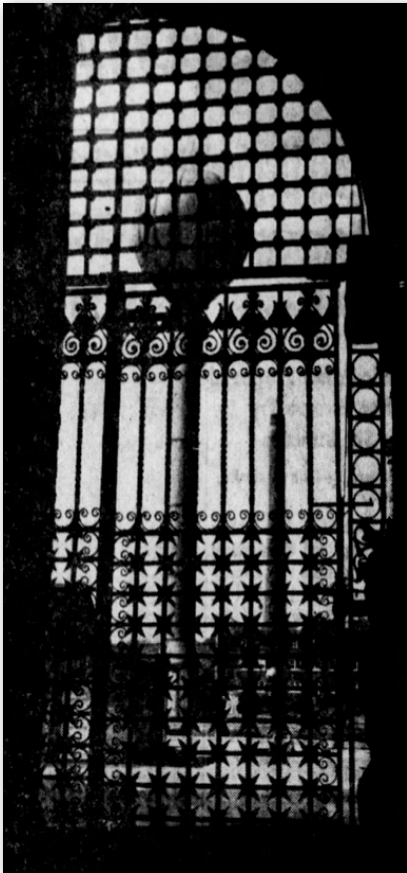
Figure 10. Porte cochere of the Warden's Residence and Offices, 1966, looking north, showing one of the ornate iron gates that originally created a secure sally porte. The porte cochere and gates were removed sometime after 1983 (Pittsburgh Press, 28 November 1966).
