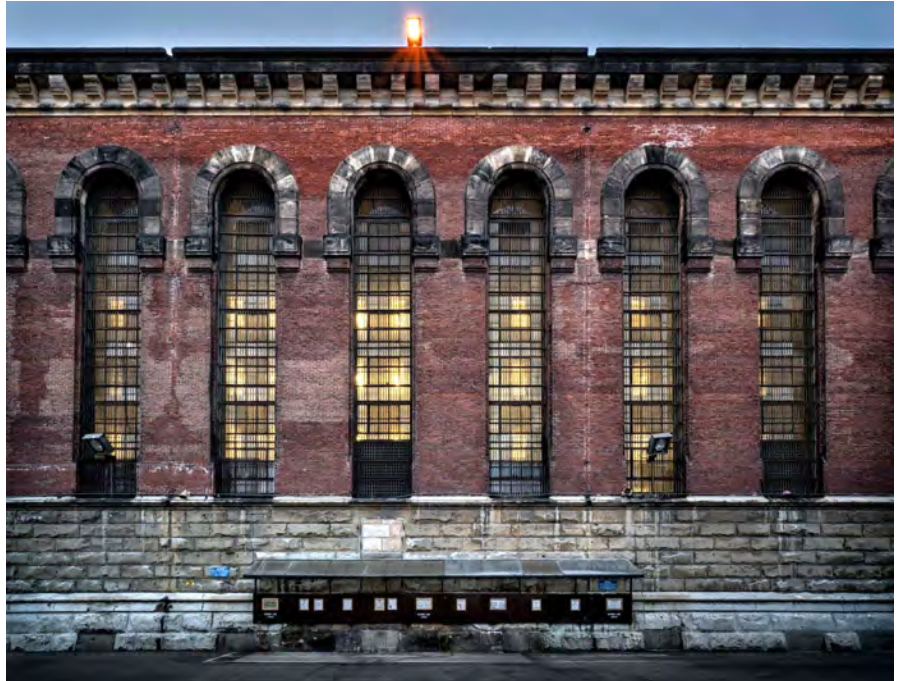
Photo 14. Main Penitentiary Building, North Wing, east facade of Housing Unit E, looking west, showing the battered stone base of the wall with arched windows and brick walls above topped by a cornice of stone modillions. Only the east facade is finished in brick; the others are clad in stone.
