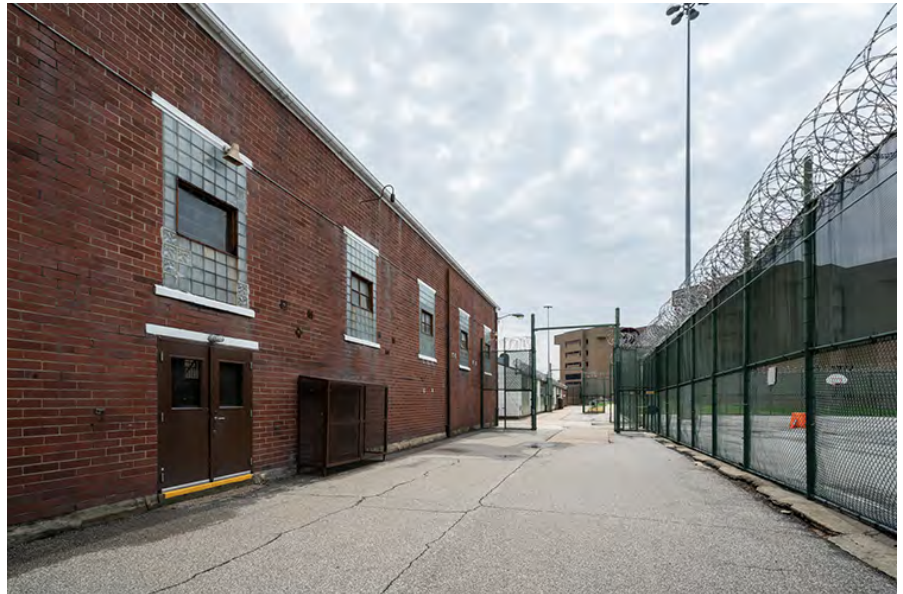
Photo 57. Gymnasium, west facade, looking southeast.
