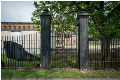
Photo 92. Cast and wrought iron gate, west side of Historic Front Yard, looking east, with the Warden's Residence in the background.
