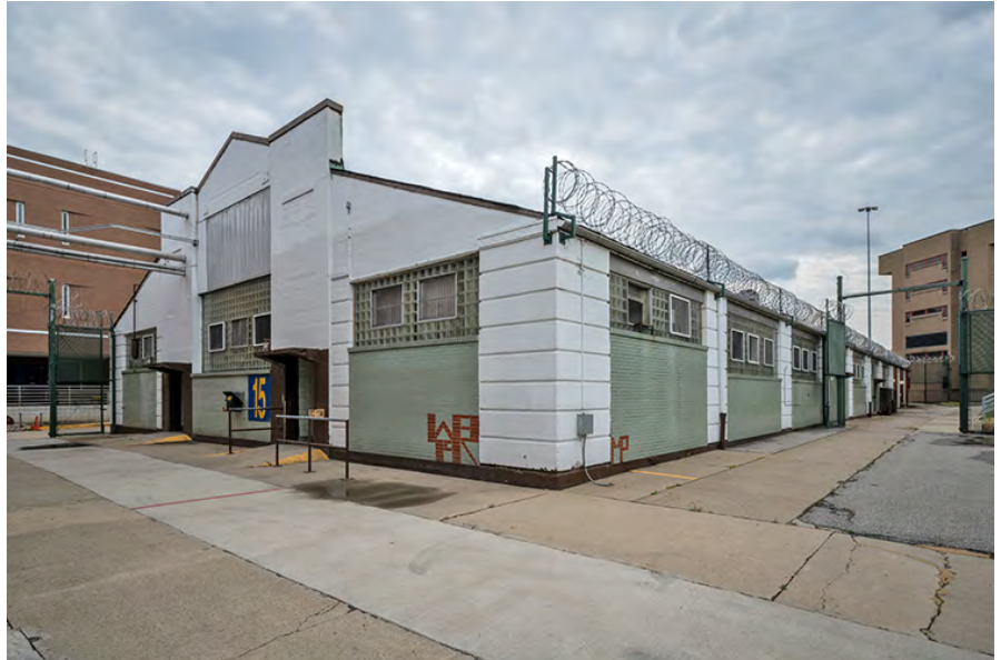
Photo 52. Dining Hall, looking southeast, showing the primary entrances to the building (left).
