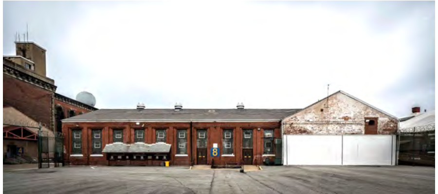
Photo 38. Auditorium/Dietary Storage Building, looking north from the Main Yard.
