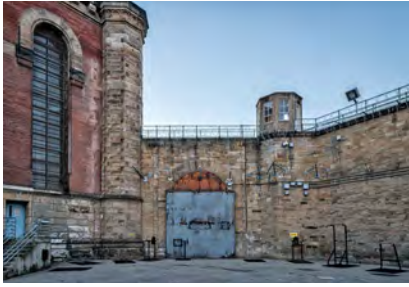
Photo 87. Northwest gate (no longer in use), looking west from within the Secure Perimeter, showing Tower 1 atop the wall.
