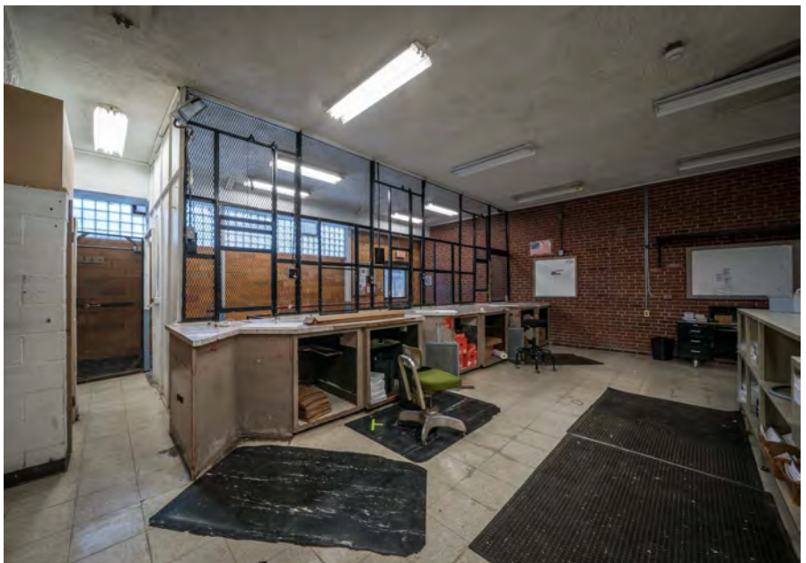
Photo 44. Services Building interior, south end, looking northwest, showing the Commissary area.
