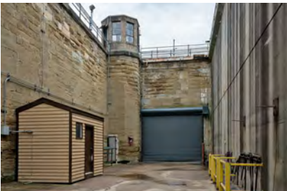
Photo 101. Guard station in Sally Port, looking west.
