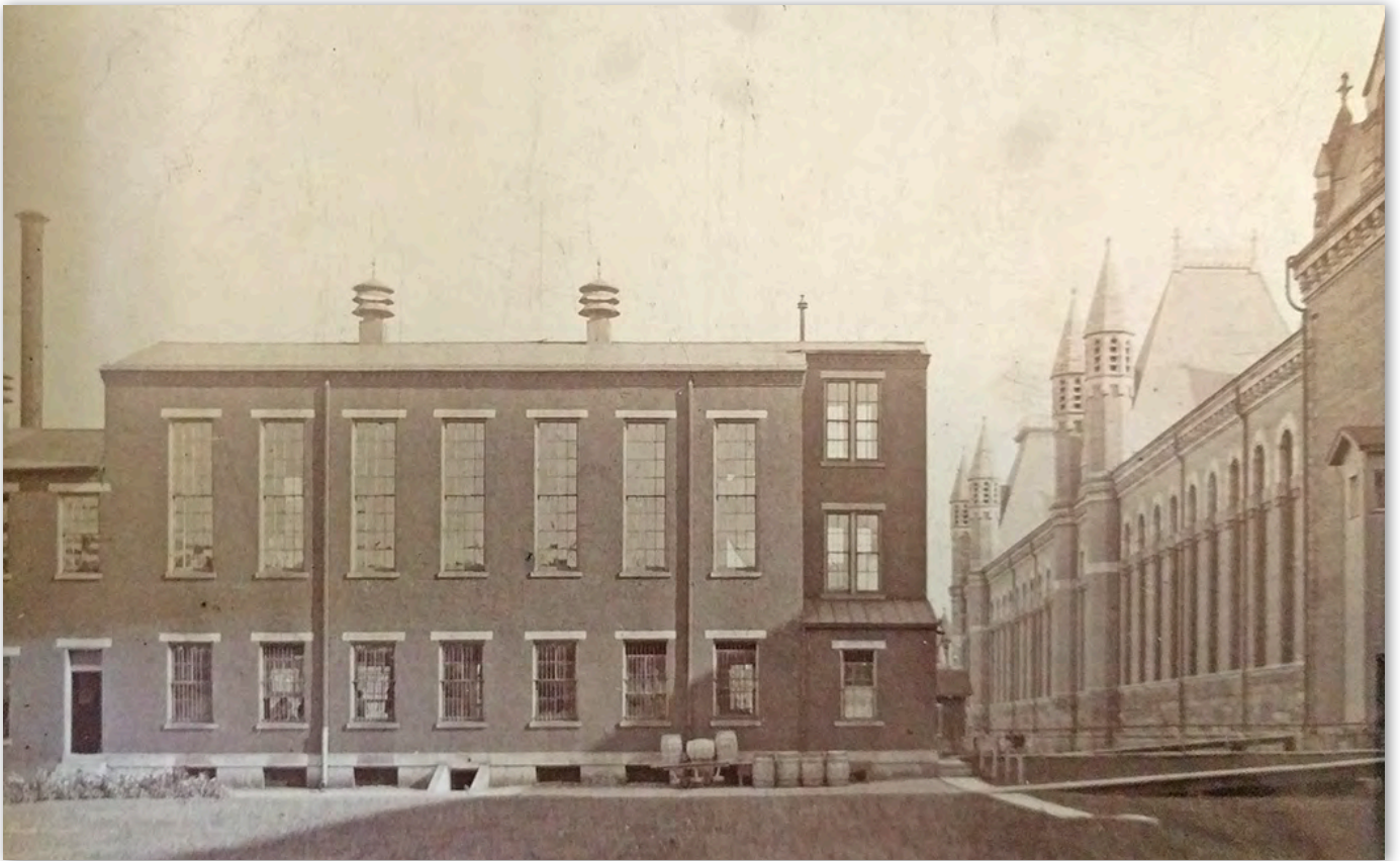
Figure 76. Ca. 1890 photo showing the East Wing of the former House of Refuge that Butz incorporated into his design. At the time of this photo, the main block of the House of Refuge has been demolished, leaving a gap between the East Wing and Main Penitentiary Building. By 1893, the stair tower (right end of East Wing) was removed and a connector was built joining the East Wing and the Rotunda (PA State Archives).
