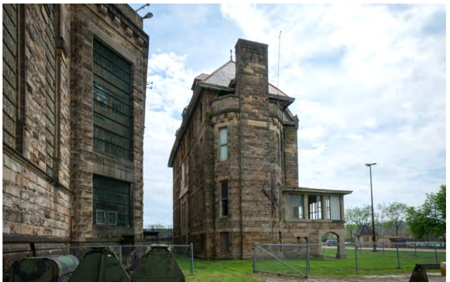
Photo 9. Warden's Residence, north facade, looking south, showing the narrow gap between the house and the Main Penitentiary Building. Also visible is one of the three-story, octagonal bay windows with integral end chimney.
