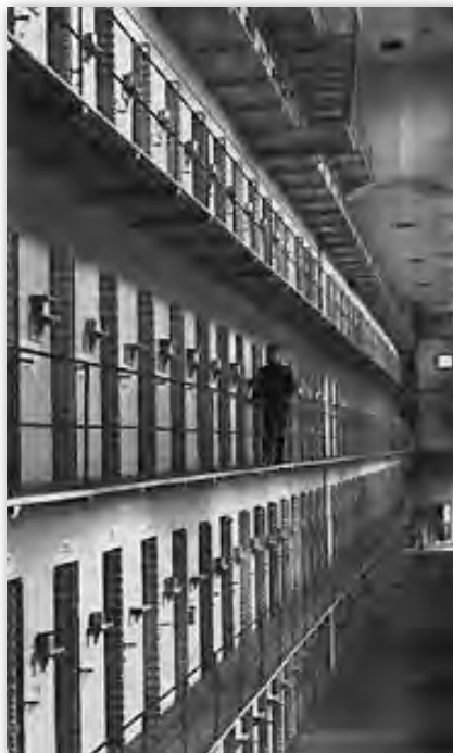
Figures 117 (bottom left) and 118 (bottom right). Photograph of Auburn cell block interior ca. 1910 on the left and Western Penitentiary cell block in 1897. A comparison of the cell blocks show how clearly the Western Penitentiary design was based in the Auburn system. Western Penitentiary, however, was built in a much more ornate manner, as shown in the elaborate cast-iron balcony brackets. This cell block design is a major departure from the plan of Eastern Penitentiary and the first Western Penitentiary in the Allegheny Commons (left: New York Correction History Society; right: Mylin, State Prisons, Hospitals, Soldiers’ Homes).
