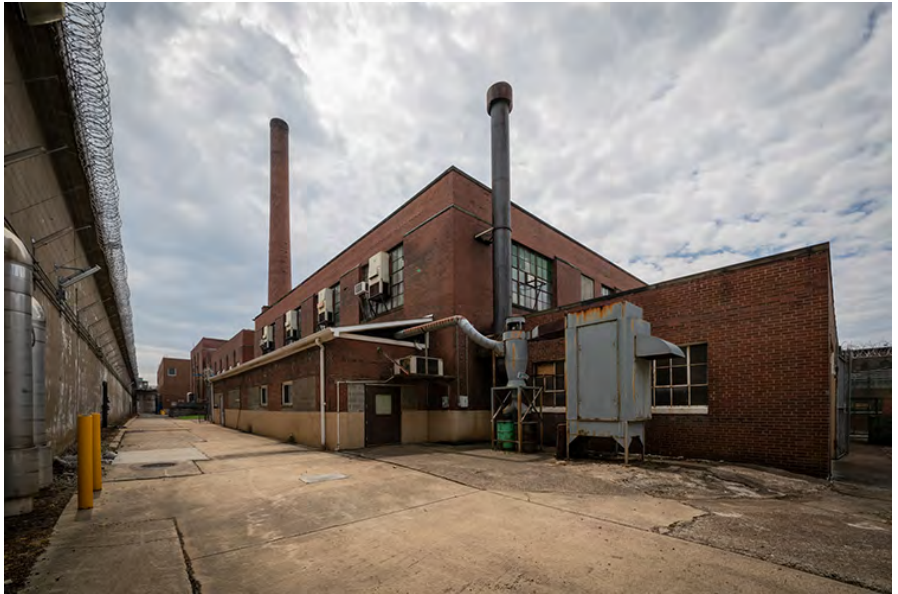
Photo 81. Maintenance Shops/Office Building, looking southwest, showing the Maintenance Repair Building (23, at left) and the Maintenance Welding Shop (29, at right).
