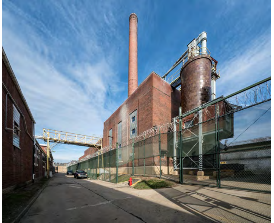
Photo 78. Exterior of Power House (right) and Boiler Plant (connected at left), looking northeast, showing the elevated site and foundation that aimed to keep equipment above flood waters.
