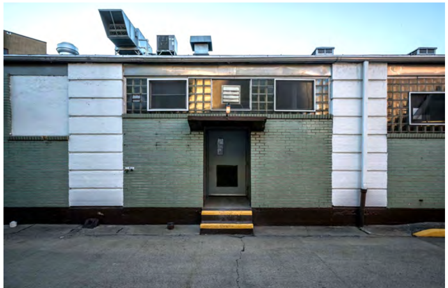
Photo 53. Dining Hall, east facade, looking west, showing a side entrance and typical building materials, such as mint green glazed brick, painted concrete piers and glass block.
