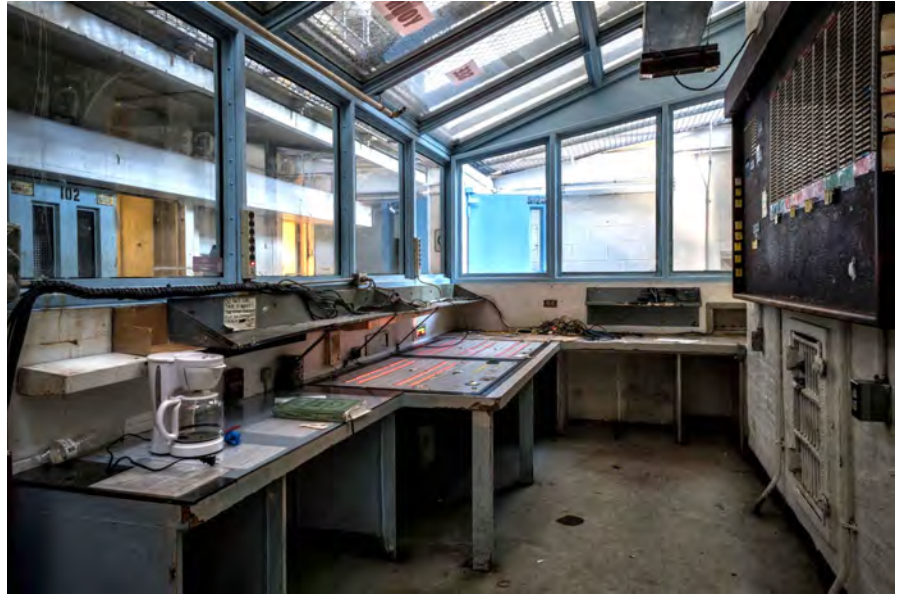
Photo 25. Main Penitentiary Building interior, Housing Unit C, first floor, looking north, showing a typical guard station with its impact-resistant glass windows and ceiling. On the table in the center is a control panel that allowed guards to remotely operate all of the cell doors.
