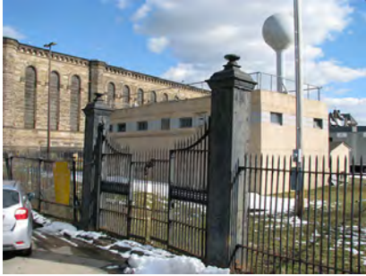
Photo 91. Cast and wrought iron gate, north side of Historic Front Yard, looking southeast (Jeff Slack).
