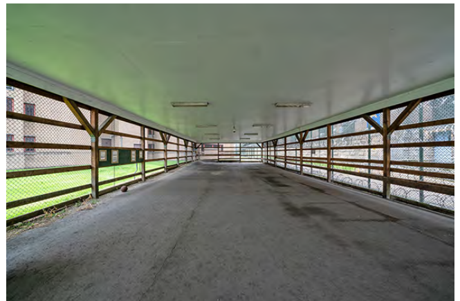
Photo 69. Exercise Pavilion interior, looking south.
