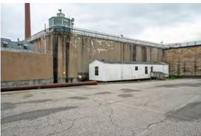
Photo 102. Corrections Emergency Response Trailer, looking southwest.
