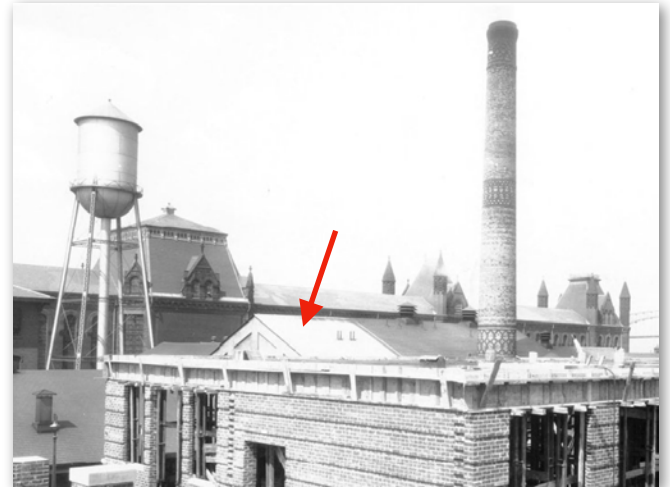
Figure 47. Detail from a ca. photo, looking northwest, showing construction of the old hospital in the foreground and the new south addition to the Gymnasium. Note that the 127-foot chimney of the old electric plant has not yet been removed (University of Pittsburgh Archives).
