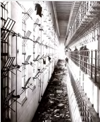
Figure 19. This photo, taken after riots in 1953, shows the mechanical operators that allowed multiple sashes to be opened and closed from the floor (Pittsburgh Sun Telegraph).
