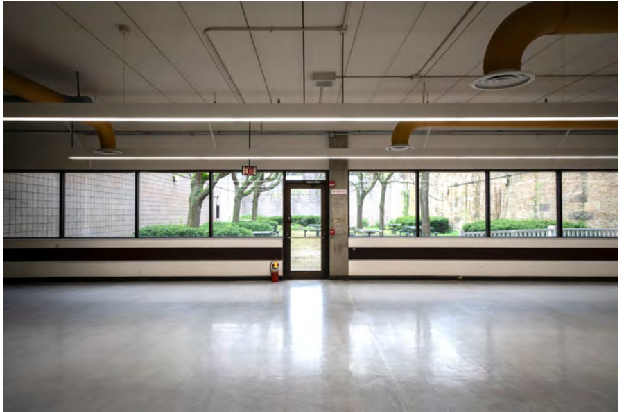
Photo 36. Administration and Visitors Complex interior, first floor, looking south, showing the visitor day room with courtyard beyond.
