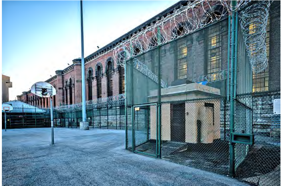
Photo 70. Inside Pump House (right), looking southwest.
