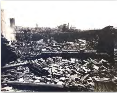
Figure 31. Remains of the historic East Wing, looking east, after rioting inmates burned down most of the buildings in the north half of the Secure Perimeter in 1921. The current building was rebuilt on this site (PA State Archive).
