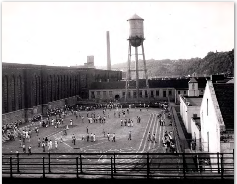
Figure 104. 1962 view of the SouthYard. The yard became considerably smaller after the construction of housing units A&B in 1985. The Chapel, School, and Female Ward, which bordered the Yard to the right, were also demolished in the 1980's (Pittsburgh Post Gazette, 1962).
