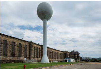
Photo 103. Water tower, looking southeast.
