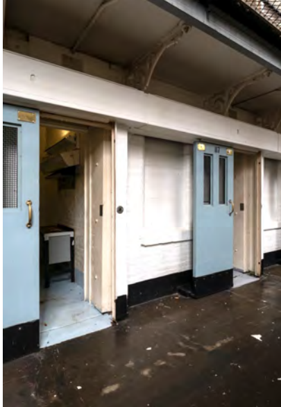
Photo 20. Main Penitentiary Building interior, Housing Unit C, looking east, showing a typical original window opening into a cell (center) that was filled with concrete block ca. 1983.
