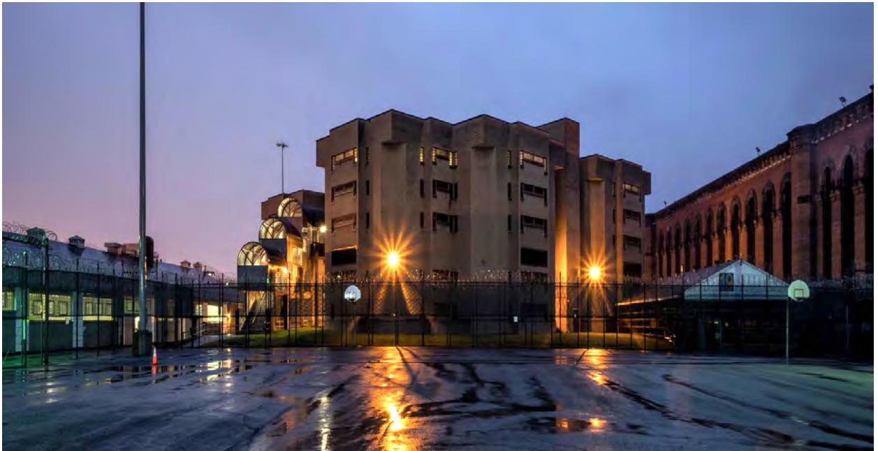
Photo 29. Housing Unit B (6), looking south from the Main Yard.
