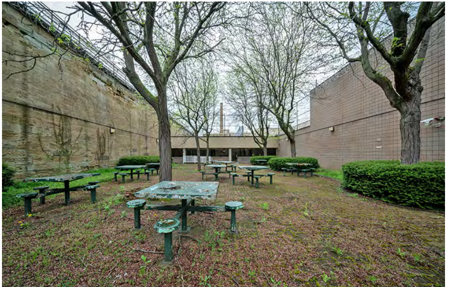
Photo 37. Administration and Visitors Complex, Visitors Courtyard, looking north, showing the original west wall of the penitentiary (left) and the visitor day room in the background.
