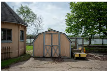
Photo 97. Shed adjacent to Guard Station (22), looking west.
