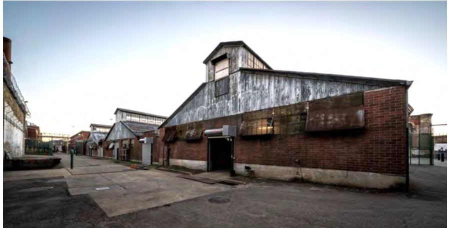
Photo 47. Correctional Industries Shop Building, looking southwest, showing (from right to left) the Welding Shop (13), the Metal Shop (12) and the Tag Shop (11).
