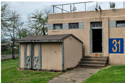
Photo 96. Shed outside Sewage Pump House, looking northwest.
