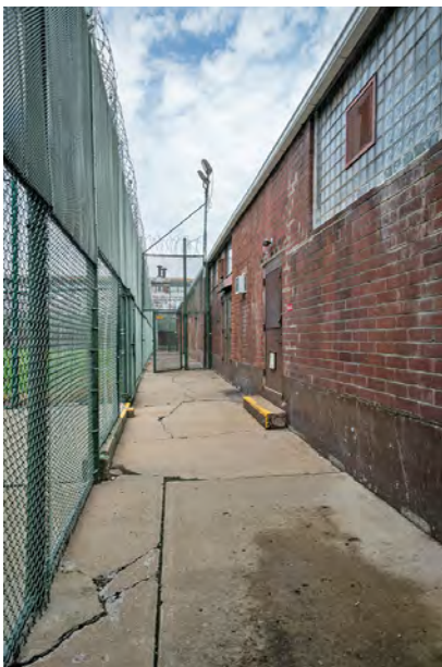
Photo 43. Services Building, west facade, looking north.
