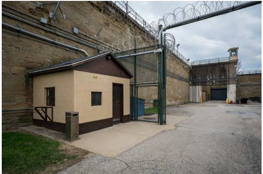
Photo 74. Scale House exterior, looking southeast.
