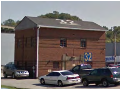
Figure 6. Maintenance Storage Building (32), looking east, showing typical building designations used on walls and roofs (Google).
