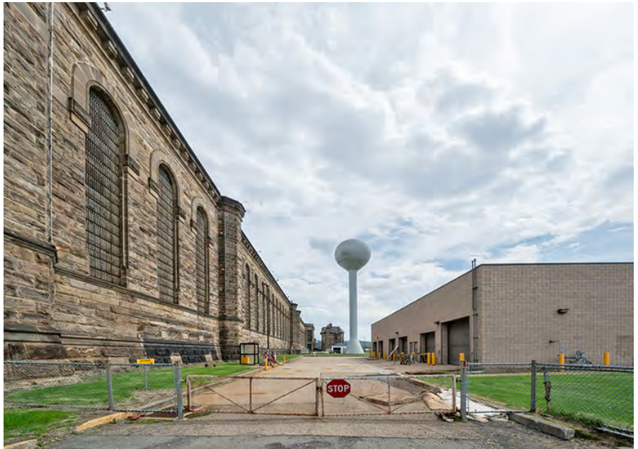
Photo 86. Vehicle Maintenance Building exterior (right), looking south.
