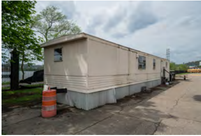
Photo 94. Modular Building (37), looking northwest.
