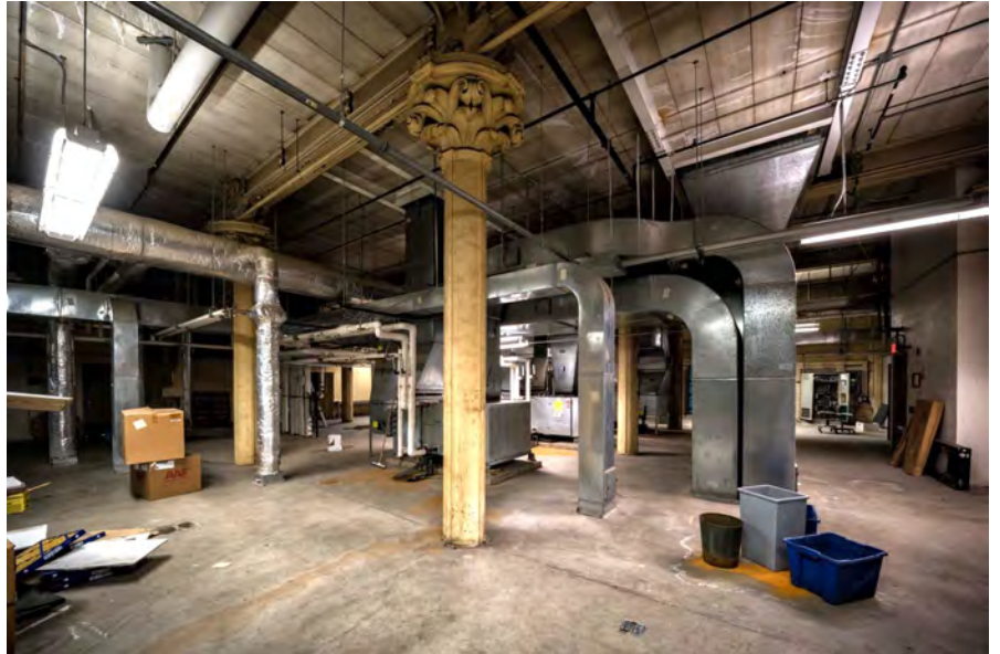
Photo 27. Main Penitentiary Building interior, fourth floor of Rotunda, looking northwest, showing the mechanical space with its floor slab that was inserted into the building in 1959 and the original cast iron columns with their decorative capitals. Similar capitals remain above the dropped ceiling on the first floor.
