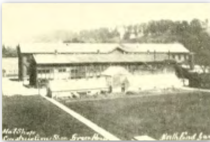
Figure 114. Photograph of the North Yard in 1897, showing several of the labor shops. From front to back, the Greenhouse, Machine Shop (also called the Construction Shop) and the Mat Factory (Mylin, State Prisons, Hospitals, Soldiers' Homes).
