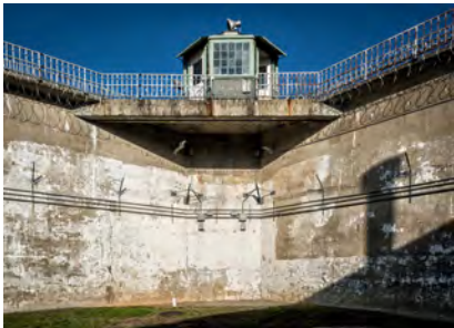
Photo 89. Tower 3, looking northeast, showing the cast concrete construction of the 1932 wall.
