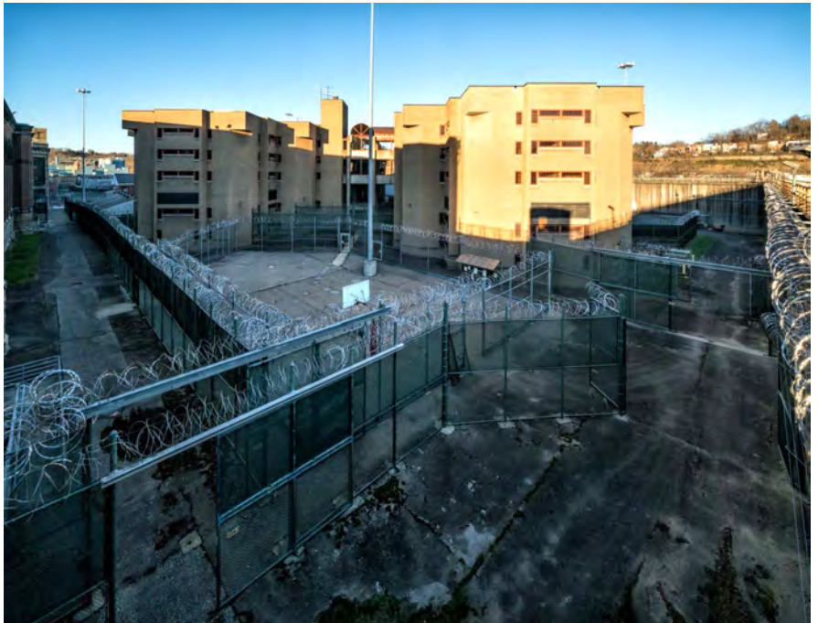
Photo 28. Housing Unit A/Building 5 (right) and Housing Unit B/Building 6 (left), looking northeast from Tower 7, showing recreation yards in the foreground.
