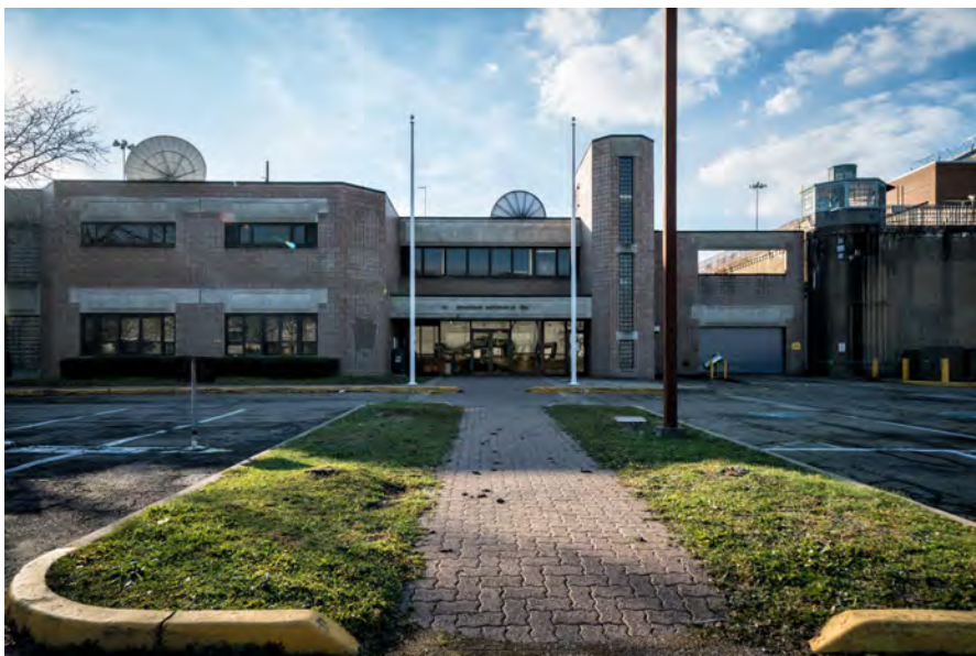
Photo 34. Administrative and Visitors Complex, east facade, looking west, showing the vehicle access door (at right) where prisoners would enter the facility for processing.
