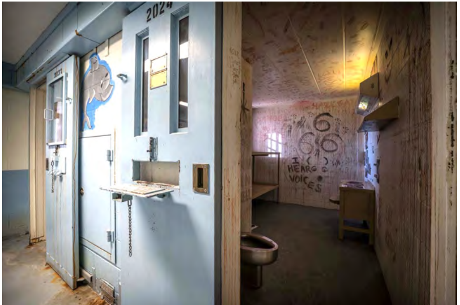
Photo 32. Housing Unit A/Building 5 interior, showing a typical second floor corridor with sliding doors and the inside of a typical cell. The fold-down panel in the center of the door was a safety feature. With the inmate inside the cell and the door locked, the inmate would place his arms through the opening. Guards could then safely attach handcuffs before opening the door. This particular unit retains considerable graffiti from its last inmate in 2017.
