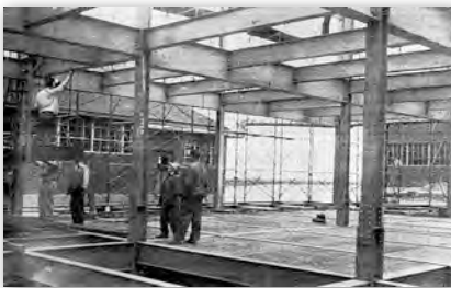
Figure 49. Construction of the Security Warehouse, 1954, showing erection of the steel posts and beams (Two Centuries of Corrections).
