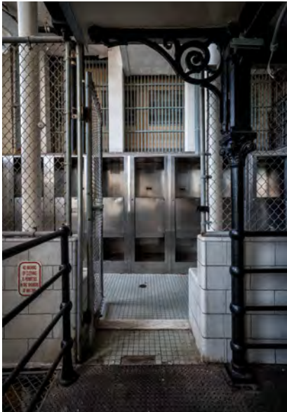
Photo 19. Main Penitentiary Building interior, Housing Unit D, looking north, showing typical stainless steel shower units.
