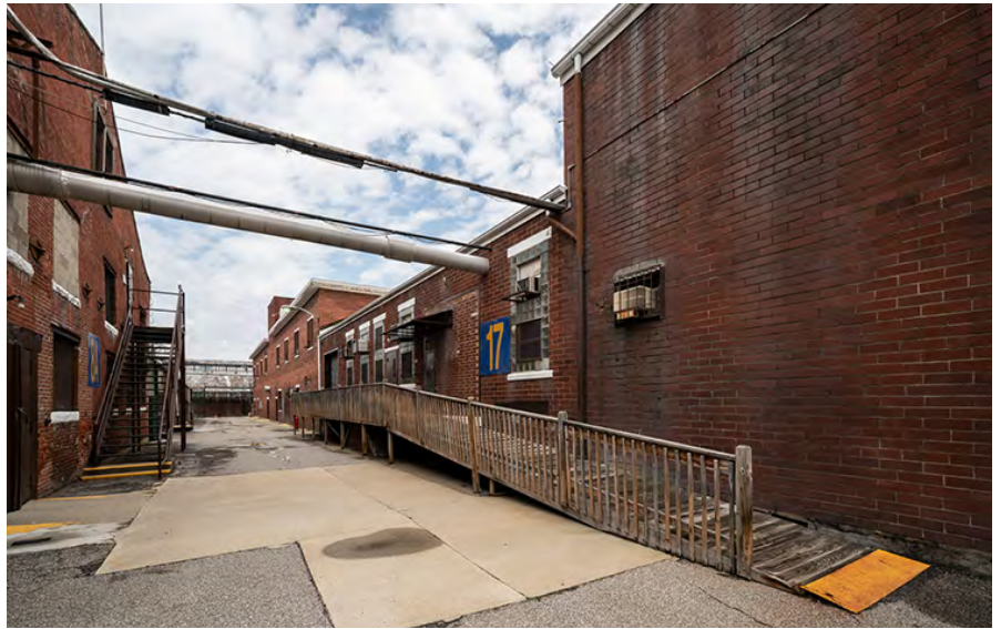
Photo 61. Maintenance Building, west facade, looking northeast.
