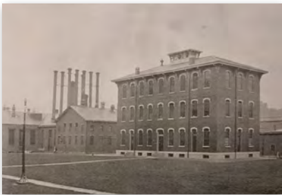
Figure 30. A view from the Main Yard in 1905 looking northeast, showing the L-shaped East Wing (at left), which housed the Kitchen, the Boiler House with its ten smokestacks, and the Bake House. To the right is the Hospital (PA State Archives).
