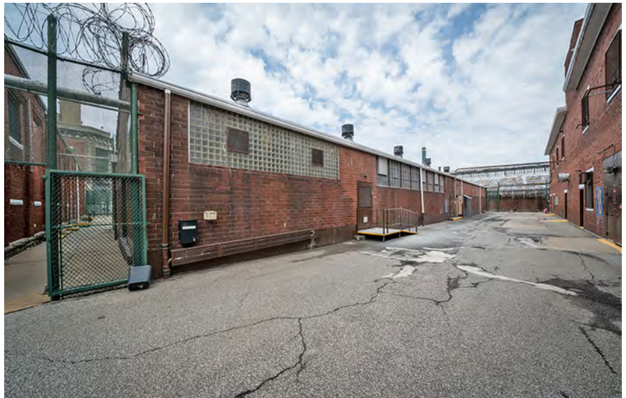
Photo 42. Services Building, east facade, looking northwest.
