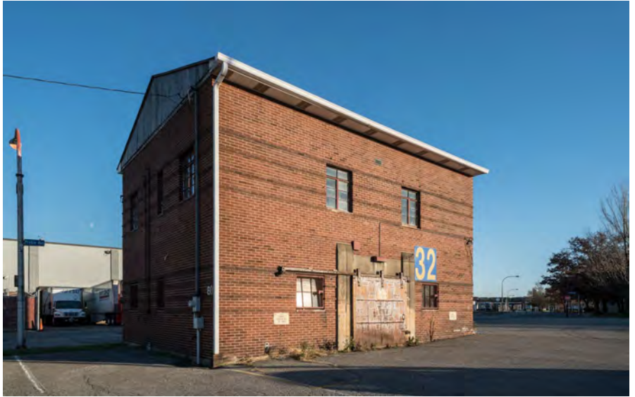
Photo 85. Maintenance Storage Building, exterior, looking southwest.
