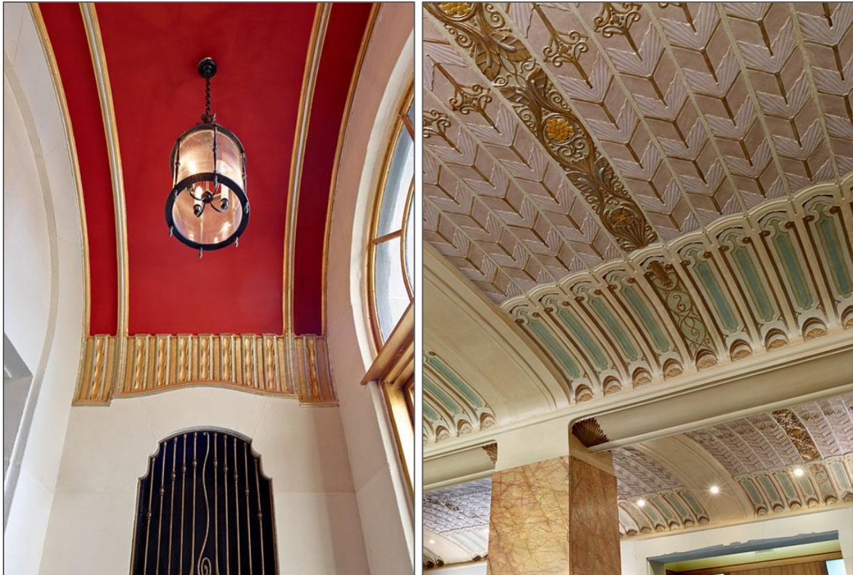
Above: Details of the lobby ceilings of the Rittenhouse Plaza after plaster restoration, decorative painting and gilding to match the historic, c. 1928 finishes
